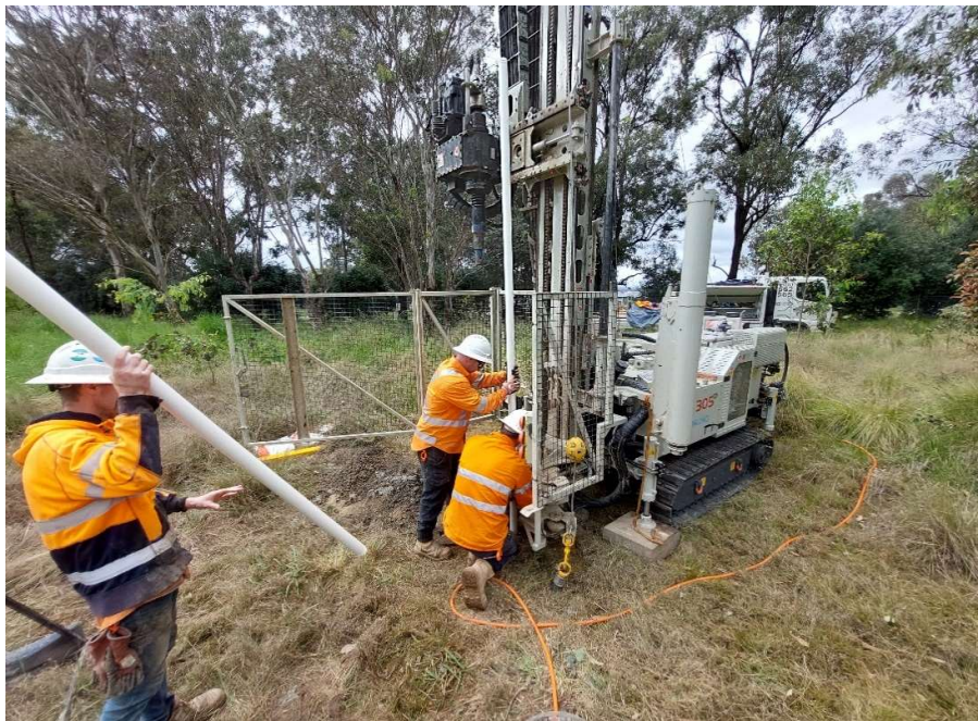
Photo 8 : Typical piezometer installation process
